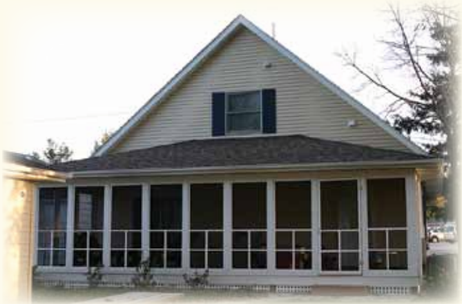
In-town cottage back porch, Spring 2007
